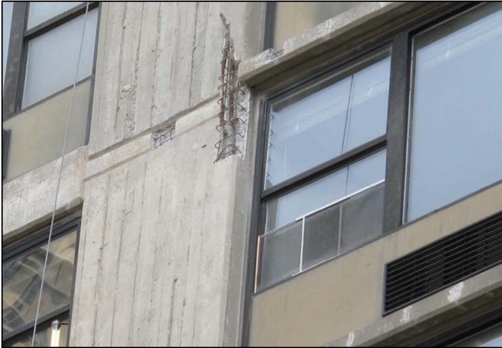
Representative example of façade maintenance in progress at Site
