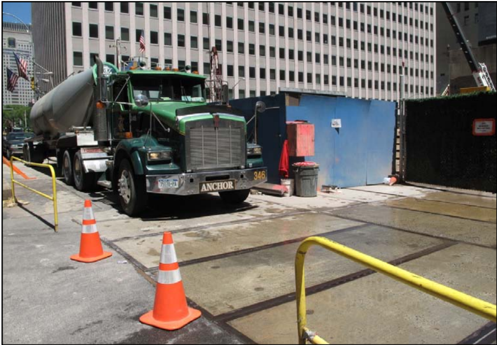
Tanker truck operating transfer pump adjacent to Site entrance
