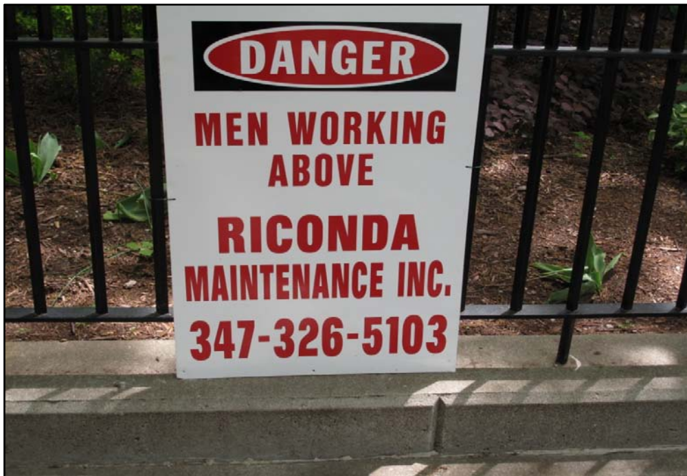
Warning sign posted adjacent to work area
