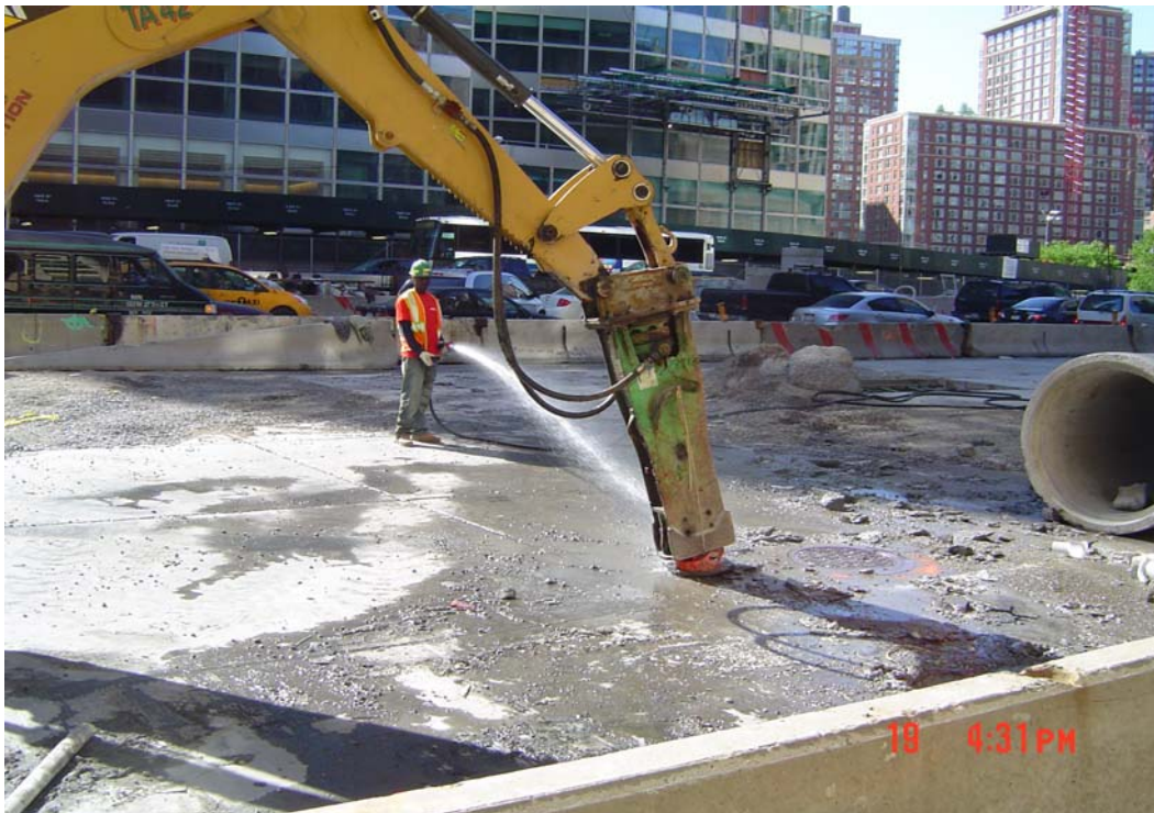
Excavator operating on 9A between Barclay and Murray
