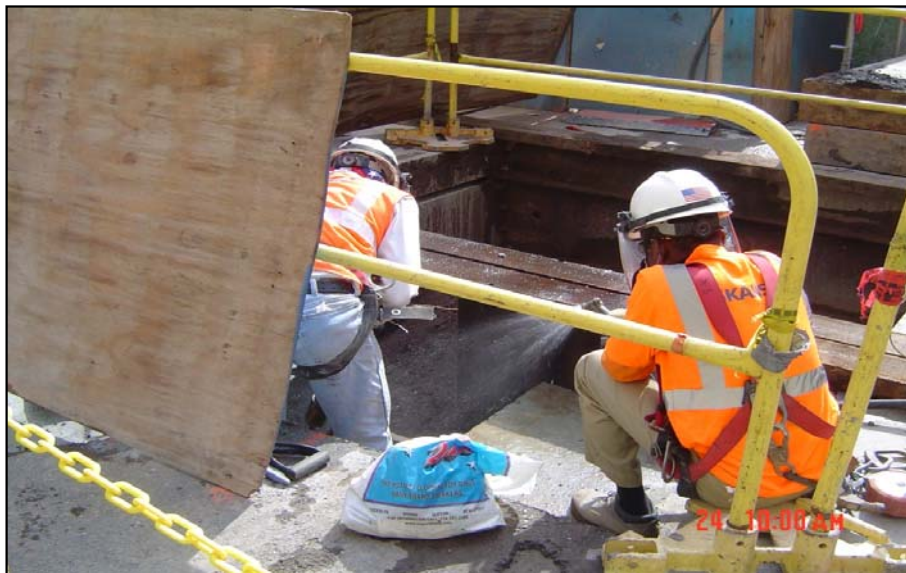
Construction personnel operating a pneumatic hammer at front entrance along Broadway.
